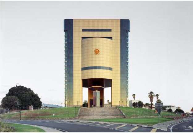
07_Independence Memorial Museum under Construction Windhoek, Namibia, 2013 © CHE Onejoon
