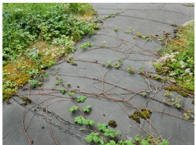
06 Site No. 11: Rhydymwyn, Flintshire © Dara McGrath
