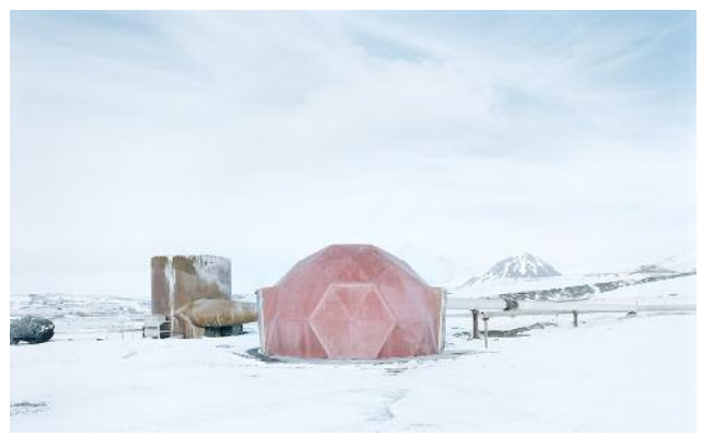
10_Krafla Geothermal Power Station, Iceland, 2021 © Gregor Sailer
