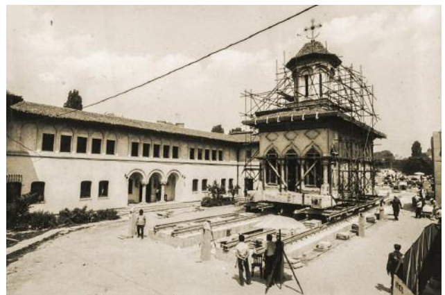
10 B_ Displacement of the Annunciation Church of the »Retreat of the Nuns«, Bucharest 1982 Courtesy Dr. Ing. Eugeniu Iordăchescu
