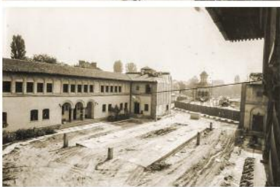
10 A_ Displacement of the Annunciation Church of the »Retreat of the Nuns«, Bucharest 1982 Courtesy Dr. Ing. Eugeniu Iordăchescu
