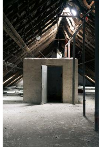
10 A Penthouse in the Making (At Work) , 2020 © Samet Durgun
