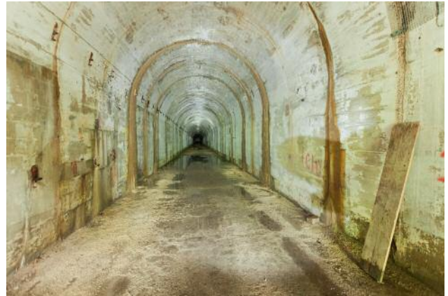
02 Site No. 11: Rhydymwyn, Flintshire © Dara McGrath
