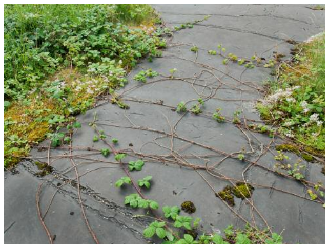
06 Site No. 11: Rhydymwyn, Flintshire © Dara McGrath
