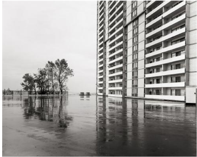
10_ North Pointe Apartments, Cleveland, 200 © Lynn Whitney
