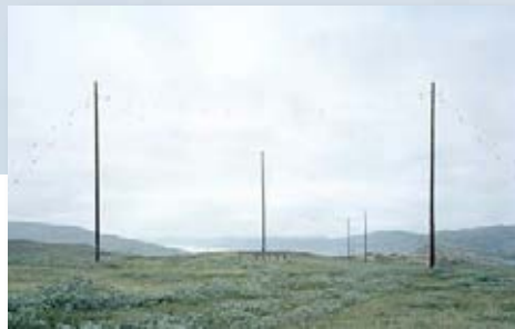
Radio Installation, Tacan, Greenland, 2019
