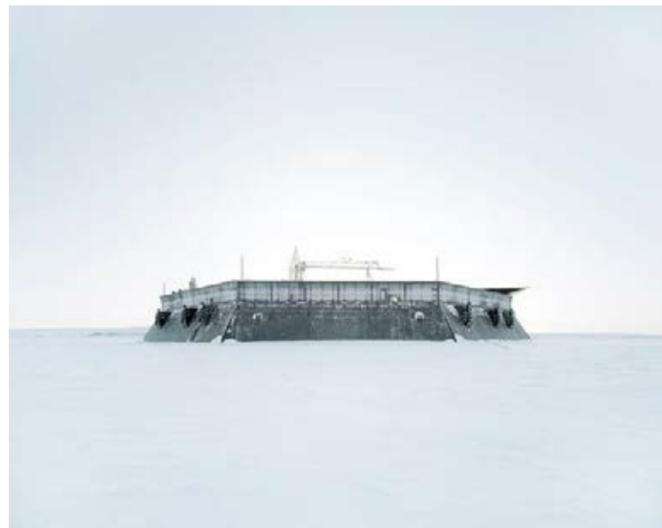
Caisson-returned Steel Island, Tuktoyaktuk, Northwest Territories, Canada, 2020
